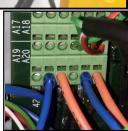
6 - The hopper sensors are connected to S1 and S2
